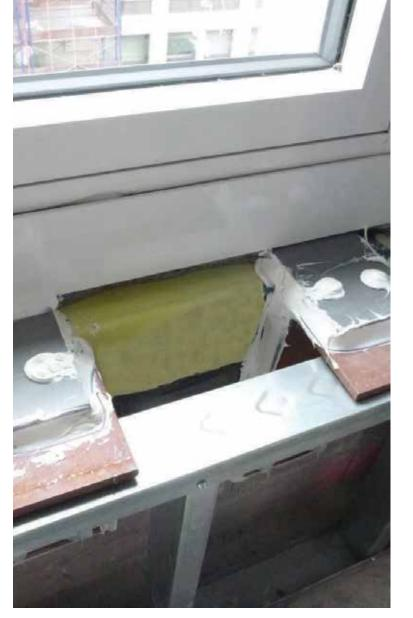
An example of highefficiency detailing, where a thermal break is provided at point transmittances, such as metal-to-metal connections. one in which more days are spent heating the building than cooling it. For example, Boston is in a heating climate, while Miami is in a cooling zone.
