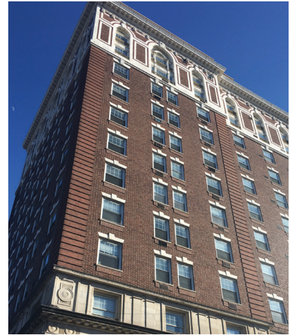
▲ Substitute materials addressed severe deterioration and weight concerns at this terra cotta cornice.
