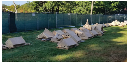
▲ Despite the owner’s proactive order of replacement terra cotta for deteriorated gables, when units were unpacked and inventoried, some were missing (left & top). Lead times for terra cotta were too long, so polymer-resin composite, carefully matched (center), filled in the gaps (right).
