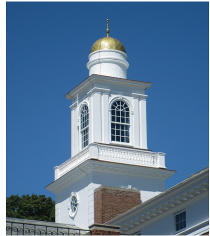
▲ Choate Rosemary Hall, Mellon Library, Wallingford, CT, Cupola Renovation, with Custom-Milled Cellular PVC in Place of Wood.
