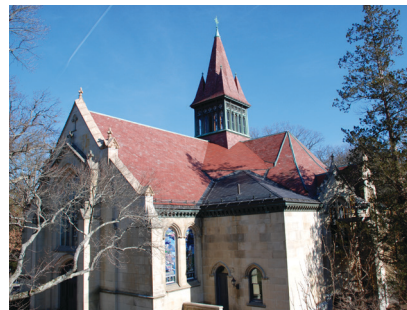
▲ Wellesley College, Houghton Chapel, Wellesley, MA, Roof Coping Replacement Using Cast Composite Resin for Missing Terra Cotta.
