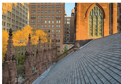
▲ Asphalt shingles mimicking slate roofing.
