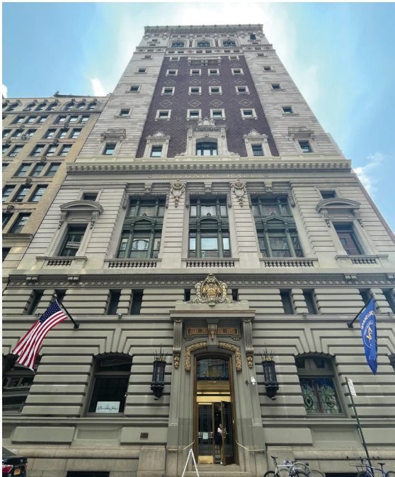
▲ Historic restoration of this Beaux-Arts tower incorporated both traditional materials and, where necessary, substitutes.
