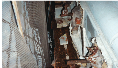
▲ Substitute materials addressed severe deterioration and weight concerns at this terra cotta cornice.
