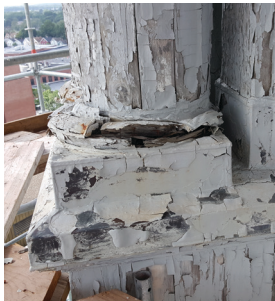
▲ Custom-milled cellular PVC in this restored cupola base resolved persistent wood rot issues.
