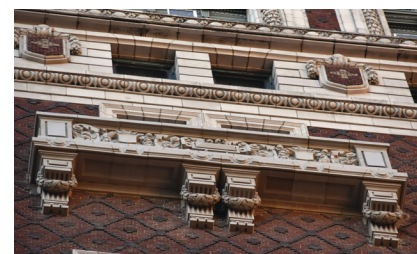
Project documents for structural rehabilitation involving substitute materials must be detailed and exacting to yield long-lasting repairs (left). At this Juliet balcony, concerns about the aging framing prompted isolated replacement of terra cotta with lightweight substitutes (right).
