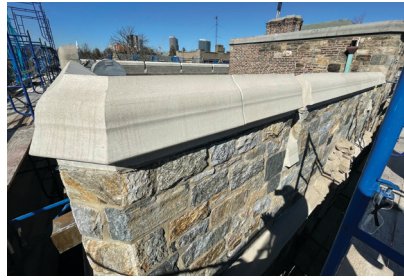
▲ Cast stone replaces limestone at a parapet.
