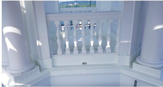
▲ Custom-milled cellular PVC in this restored cupola base resolved persistent wood rot issues.
