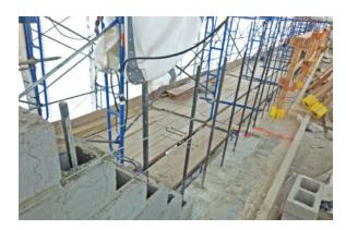
Steel bars reinforce the concrete masonry unit core of the new parapet.
