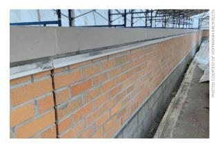
With the copings and flashing in place, the parapet is nearly complete.
