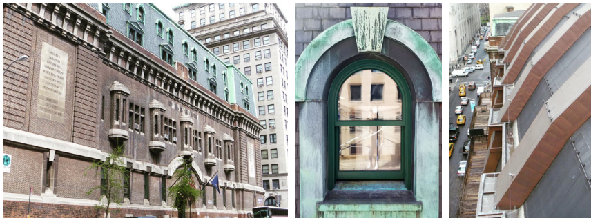
A Once automatically exempt from the New York City Energy Conservation Code, historic buildings now must comply unless they can prove that doing so would threaten historic qualities.
