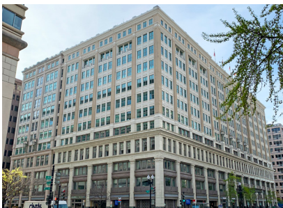
A The Homer Building , Washington, DC, Roof Replacement, Penthouse Energy Upgrades.
