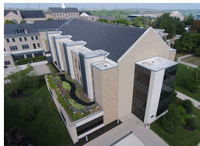
A Niagara University, Academic Complex , Niagara University, NY, Facade Replacement.
