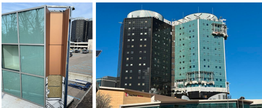
▲ Mockups (left) reveal how components such as air barriers, insulation, metal panels, vision and spandrel glass, and framing come together, identifying potential issues prior to construction (right).
