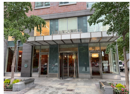
A Projection factor measures shading effect of window canopies, which dictates required SHGC.
