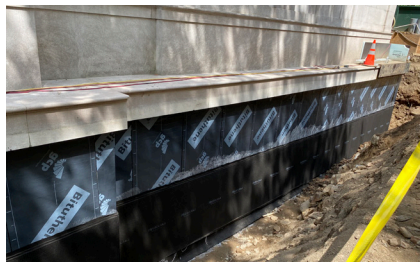
▲ Positive-side foundation waterproofing (left) is exterior; negative-side (right) is at the interior.
