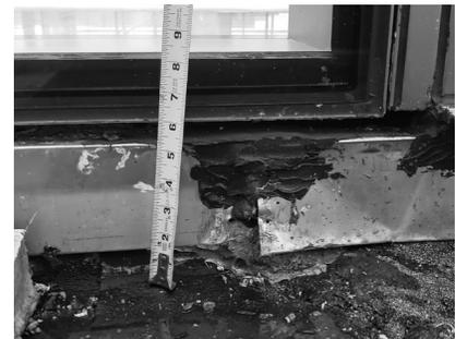
▲ Low curbs and thresholds pose a challenge when insulation height must be augmented.
