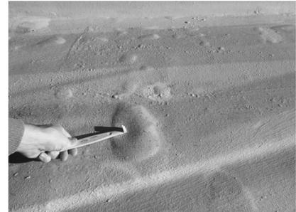
▲ Recoating an existing roof that isn't watertight won't solve moisture problems.
