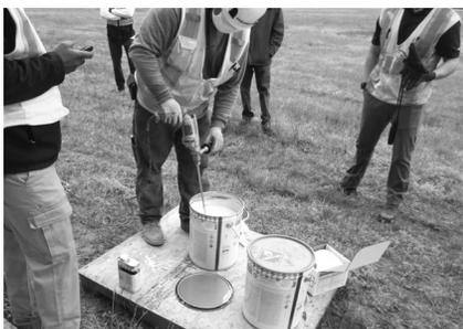
▲ Two-component reinforced liquid resin recover systems, such as PMMA, cost more and require on-site mixing (left) but provide a seamless solution for complex roof areas (right).
