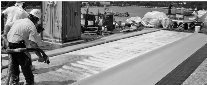
▲ Installers apply spray adhesive for a single-ply assembly during a roof replacement project.
