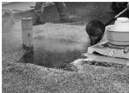
▲ Prior to installation of a recover system over an MBR assembly, loose granules in the existing cap sheet must be removed (left) or embedded in an asphalt flood coat (right).
