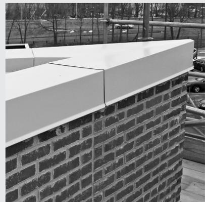
▲ Parapet copings prevent water infiltration that can migrate under the roof membrane.
