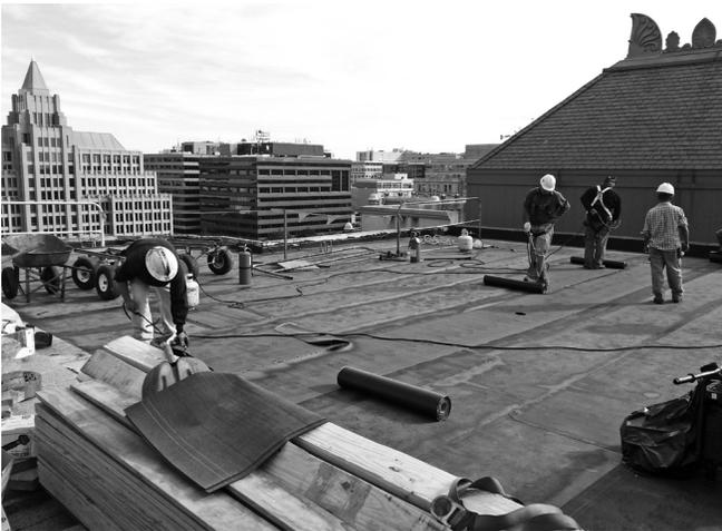
▲ Installation of a replacement modified bitumen roof (MBR) assembly provides durable long-term protection for this cultural institution.
