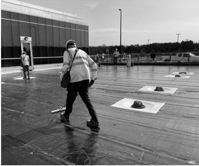
▲ Electric leak detection is a non-invasive way to pinpoint breaches in the membrane.
