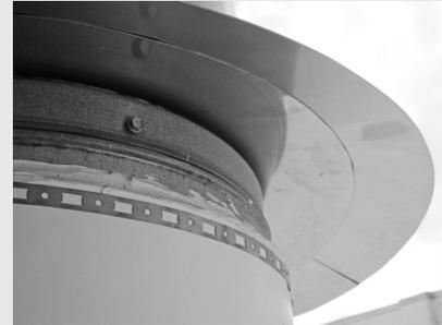
▲ Clamp rings secure the membrane around circular penetrations.
