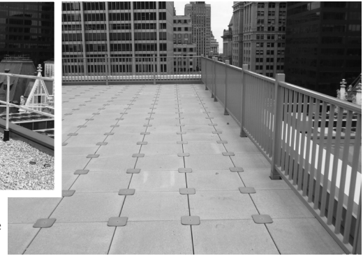
▲ For non-accessible roofs, pavers create a clean look (right) and improve safety over ballasted systems (left).
