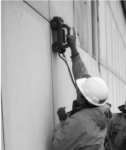
▲ Ground-Penetrating Radar (GPR) identifies anchor locations without removing panels.
