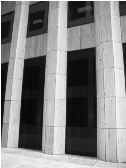
▲ New stone-cutting technology permits thinner marble panels—and brings new design challenges.
