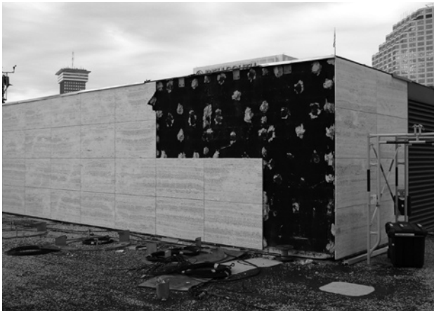
▲ Penthouse marble panel replacement in process.
