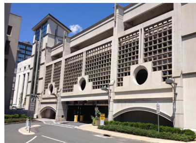
▲ State University of New York System Administration, Plaza Parking Garage, Albany, NY, Comprehensive Parking Deck Rehabilitation and Structural Consultation.
