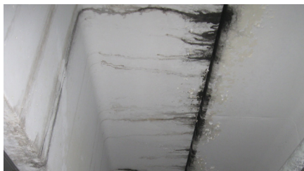
▲ Clockwise from bottom left: Soffit discoloration due to leaks, corrosion at an overhead edge spall, spalled concrete ready to fall, failed patch repair at an edge spall, and repair in progress for dissimilar metal corrosion of reinforcing bars.
