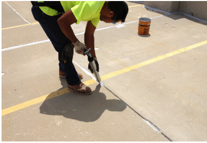
▲ Replacing sealant at a garage's top deck.
