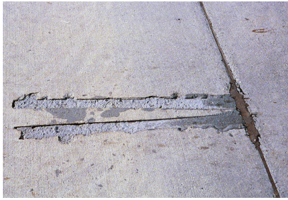
▲ Deteriorating connection repair.
