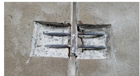
▲ Clockwise from bottom left: Soffit discoloration due to leaks, corrosion at an overhead edge spall, spalled concrete ready to fall, failed patch repair at an edge spall, and repair in progress for dissimilar metal corrosion of reinforcing bars.
