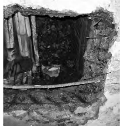
▲ A test cut into this concrete ceiling reveals wire mesh compromised by corrosion.
