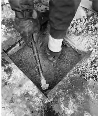
▲ Since damage to wire-reinforced floors may compromise load capacity, invasive probes require experience and planning.
