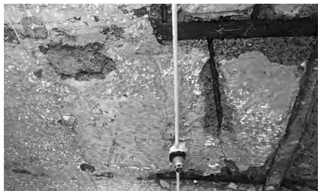
▲ With a pumice-like texture that is rough and porous, cinder concrete uses byproducts of coal as economical, lightweight, fire-resistant aggregate (left). Often, a surface of wire lath was suspended below the beams and coated with plaster to provide a finished ceiling (right).
