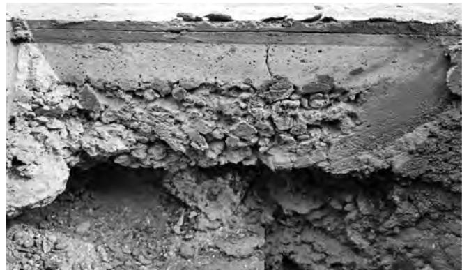
▲ Typically 1 part cement, 2 parts sand, and 5 parts cinders, cinder concrete slabs are structurally unstressed, relying on wires to carry loads.
