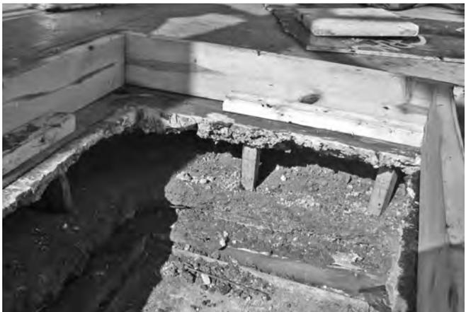
▲ Cinder concrete decks were favored in the 1920s-40s for their load capacity, fire protection, light weight, low cost, and ease of construction.
