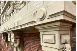
thickness of the shell. The danger of falling terra cotta merits special mention in the FISP guidelines and requires immediate stabilization.
