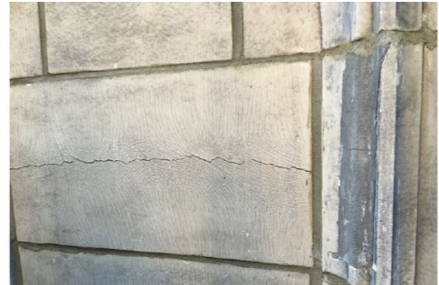
Typical glaze crazing, which compromises water penetration resistance. Cracking indicates where stress exists, often due to corrosion of anchorage. On top, an inappropriate repair is failing, as the underlying deterioration mechanism was unaddressed, and the incorrect material was used.
