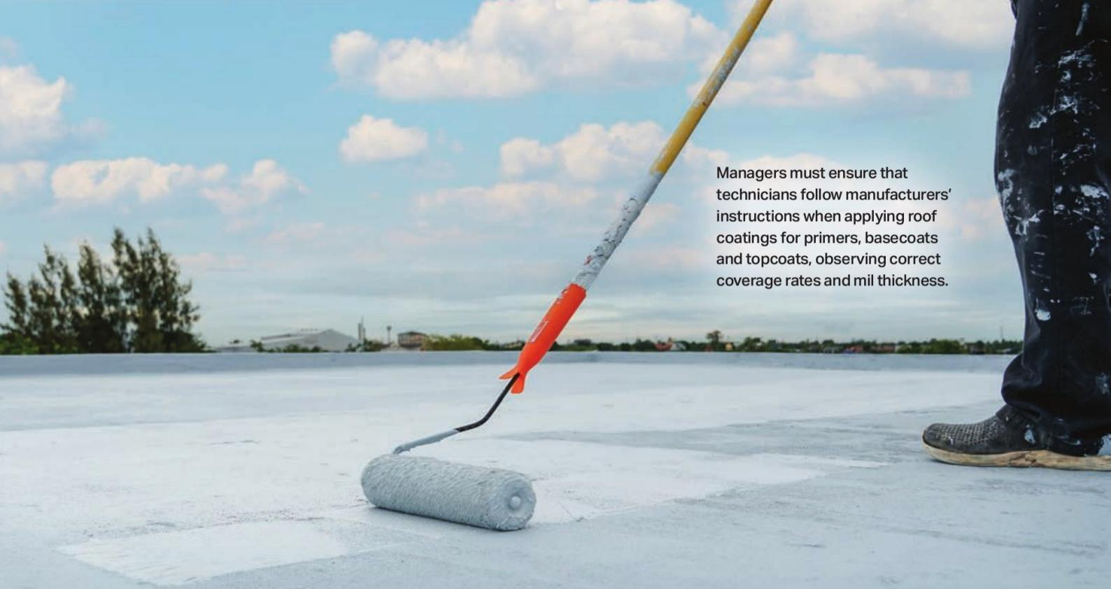
Managers must ensure that technicians follow manufacturers' instructions when applying roof coatings for primers, basecoats and topcoats, observing correct coverage rates and mil thickness.
