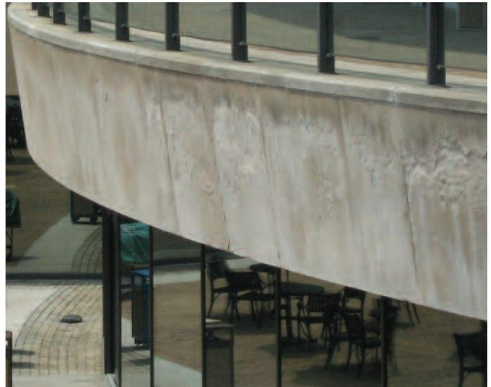
*Freeze-thaw and salt damage.*
