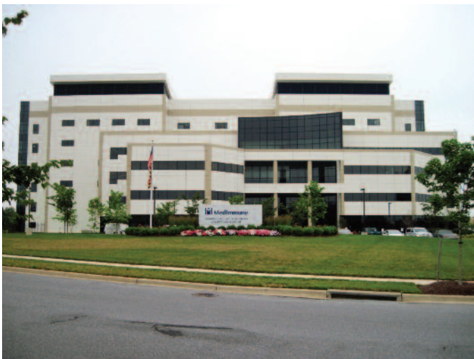
Evaluation of the coated insulated steel panel façade at this manufacturing center traced the source of recurrent leaks to incorrect installation.
