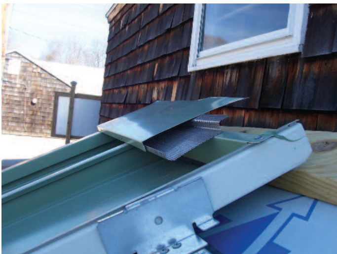
This aluminum standing-seam roof system is installed over ice-dam membrane, as well as stiffening ribs at the flat of each panel to minimize oil canning and telegraphing of structural members.
