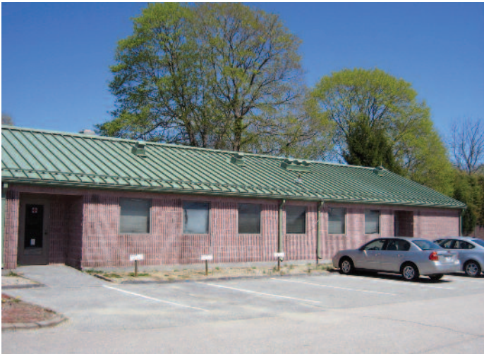
For this military training camp, standing-seam aluminum roofs with a high-performance resin coating met fast-track project demands, while offering durability in the harsh seaside climate.
