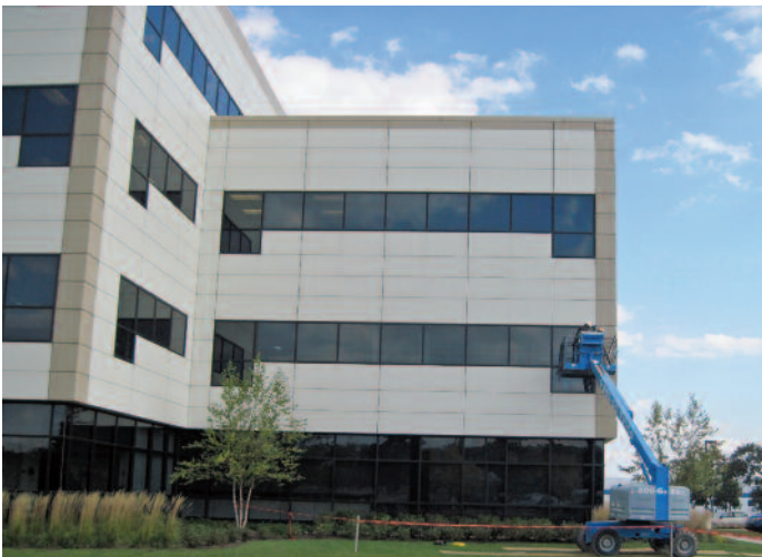
Leak investigation at this steel panel façade pointed to faulty installation practices.
