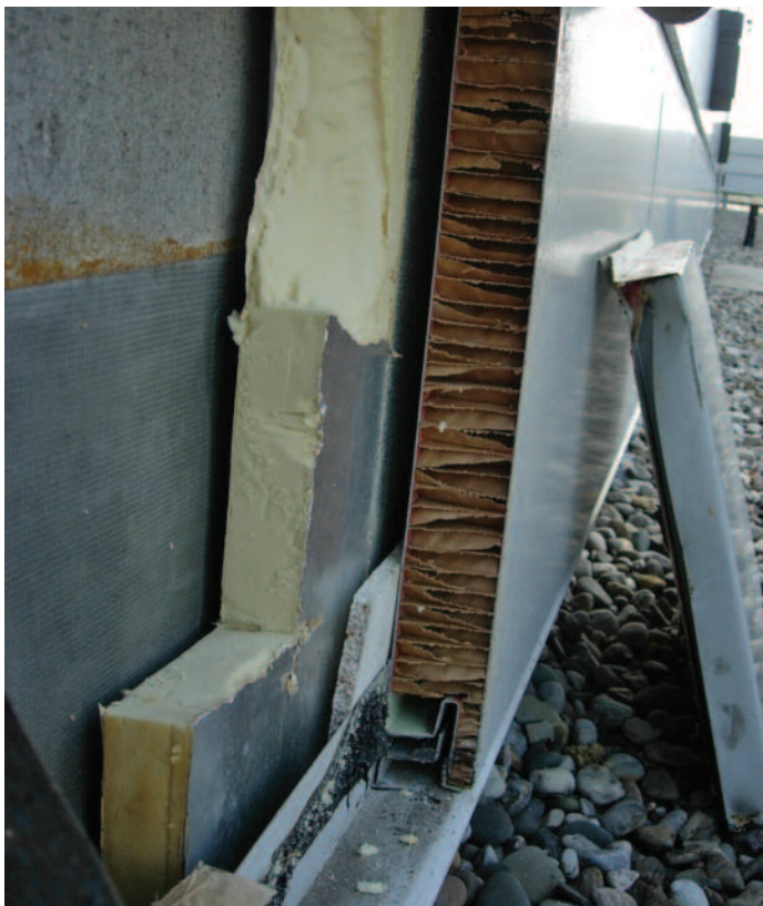
Installed in the 1990s, this metal cladding system consists of painted steel composite panels with a paper honeycomb core. Rigid insulation, inboard of the panels, provides thermal resistance.
