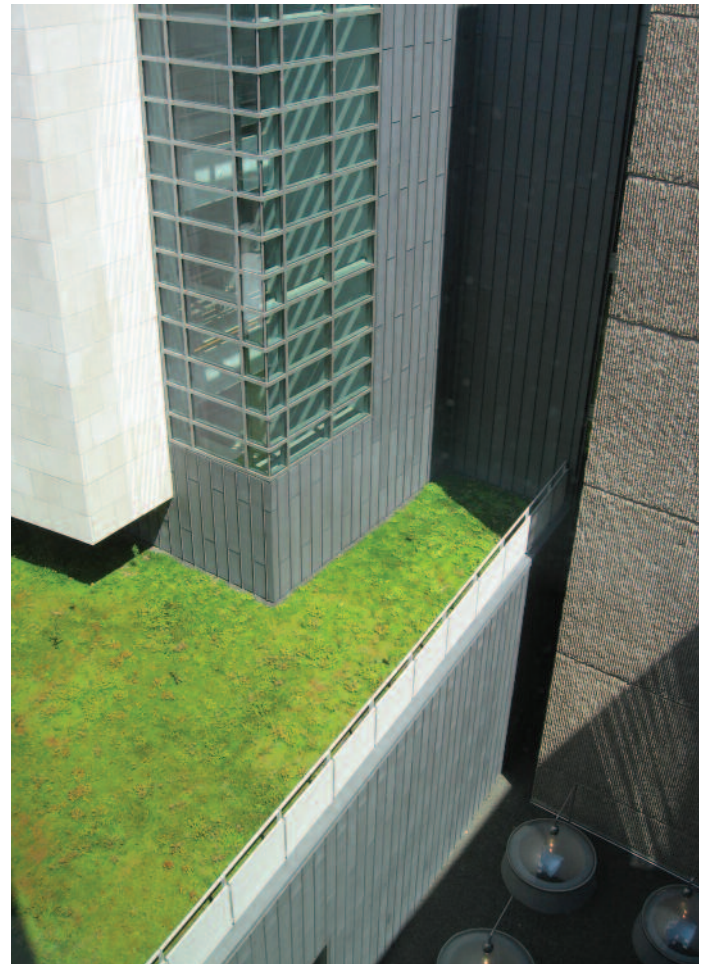
Metal façade systems come in a variety of materials, including aluminum, copper, stainless steel, and zinc, pictured here.
