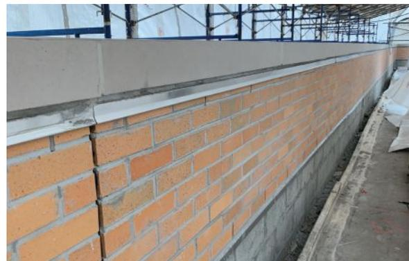
► **With the copings and flashing in place, the parapet is nearly complete.**
