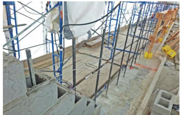
► **Steel bars reinforce the concrete masonry unit core of the new parapet.**
