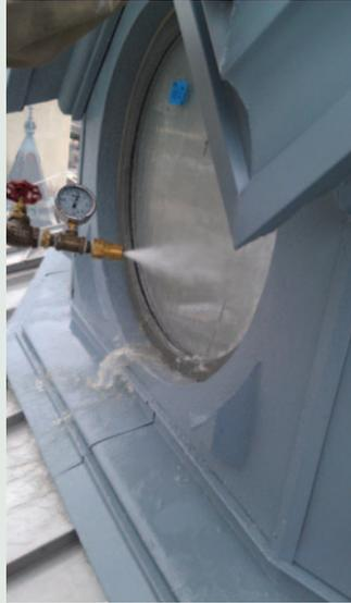
*Water test of newly installed window.*
