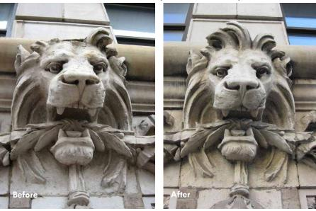
root cause of distress, using materials that are compatible with the existing terra cotta, and which do not compromise the breathability and moisture balance of the assembly. In addition, maintaining materials adjoining the terra cotta, including flashing, capping, roofing, and sealant at doors and windows, is vital to averting deterioration.
