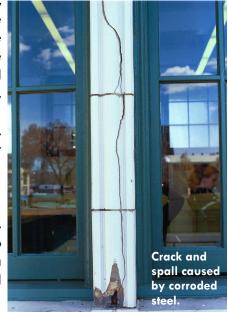
What makes embedded steel corrosion challenging to treat is that it tends to be difficult to diagnose unless it is severe. By the time symptoms are visible at the surface, corrosion is likely already advanced. Initial outward signs of metal anchoring deterioration might include staining and spalling. Total anchoring failure can result in loose terra cotta units, which are in
