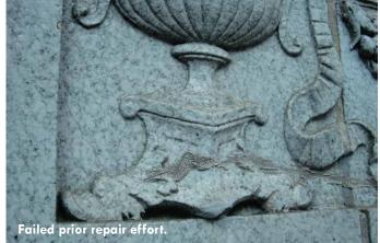
elements. Where anchoring is extensive and complex, deterioration and failure likewise tend to be more pronounced. Deterioration to terra cotta used as load-bearing masonry tends to be less severe, owing to its simple or limited anchoring system, which presents fewer opportunities for corrosion-induced cracking and failure.
