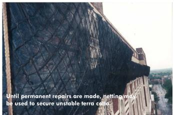
terra cotta pieces should be laid out in configuration, to confirm dimensions and colors. Where possible, replacement units should be anchored similarly to the originals.
