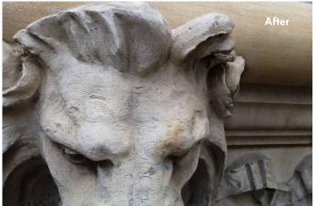
solutions may be suitable for use on terra cotta; check manufacturers' recommendations. Avoid abrasive cleaning, such as sandblasting, as well as high-pressure water or metal bristle brushes, all of which can damage glazing irreversibly.
