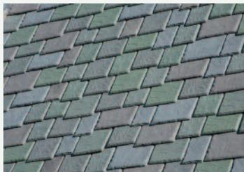
*Example of synthetic slate roofing shingles.*
