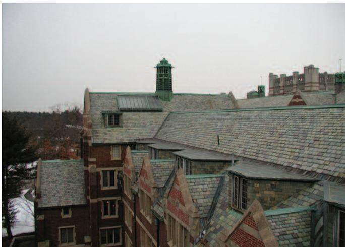
*With regular maintenance and appropriate, periodic repairs, a well-designed slate roof can last upwards of a century.*
