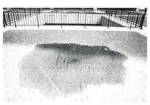
Closed joint plazas are separated into individual watersheds. Increasing the pitch of the surface immediately surrounding the drain can prevent puddles from spreading too far when drains clog, as they often do.
