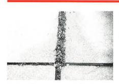
Resilient fillers were provided in this closed joint plaza to take up thermal movement, but some joints have opened over time—pointing out the need for a secondary drainage system under the plaza surface.
