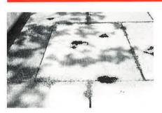
While open joint plazas have many practical and visual advantages, maintenance is important to prevent debris (in this case, pine needles) from clogging the joints and drainage system underneath.
