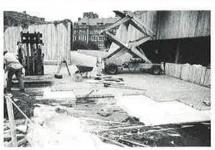
Open joint plaza slabs are relatively easily removed and replaced for inspection, cleaning, and repair. Lack of mortar joints eliminates many maintenance problems common in closed system plazas.
