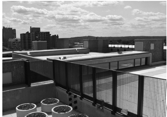
▲ Yale University, Paul Rudolph Hall (Art + Architecture Building) in New Haven, Connecticut. Roof Replacement and New Construction Consultation – Vegetative Roof and Cold-Applied MBR System with Reflective Cap Sheet.
