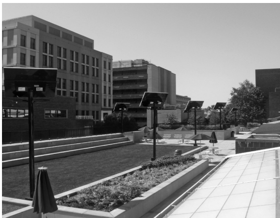
▲ New Jersey City University, Michael B. Gilligan Student Union in Jersey City, New Jersey. Roof Replacement – Intensive Green Roof and MBR System with Reflective Cap Sheet.
