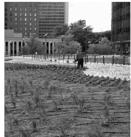
▲ Phoenix Companies Headquarters in Hartford, Connecticut. Plaza as Green Roof – Intensive Roof Garden over Offices and Garage.
