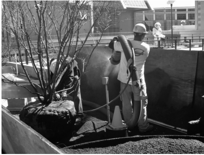
A Installation of planting medium around a large shrub on an intensive green roof.
