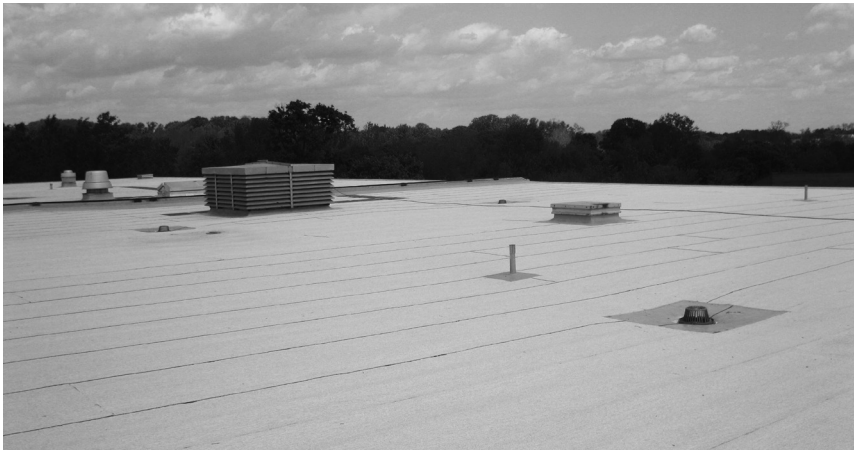
A The white cap sheet on this cold-applied modified bitumen roof assembly reflects solar radiation and disperses heat energy away from the building, keeping the interior cool.
