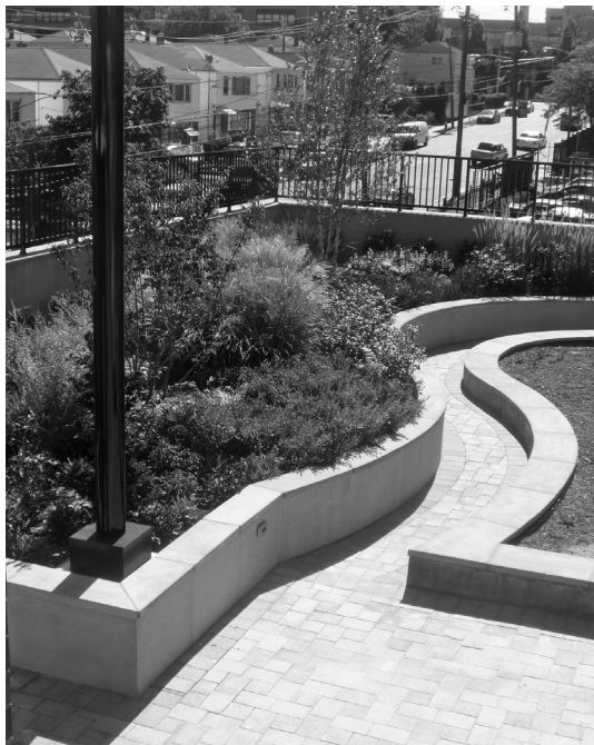
▲ Vegetative roofs can be an attractive amenity, creating a pleasing outdoor space and adding value to the building.
