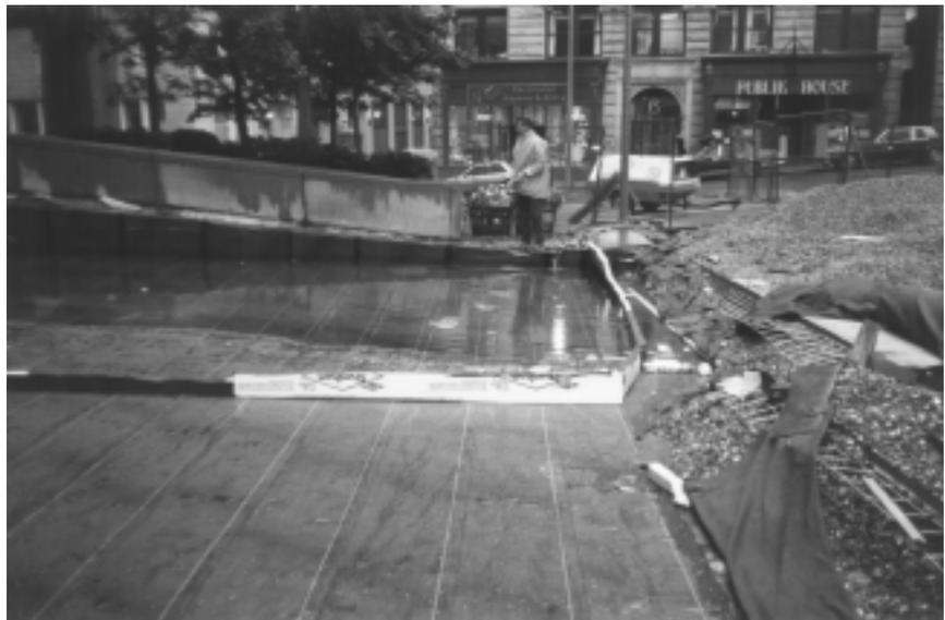
Flood testing is recommended after installation of the new waterproofing membrane.
