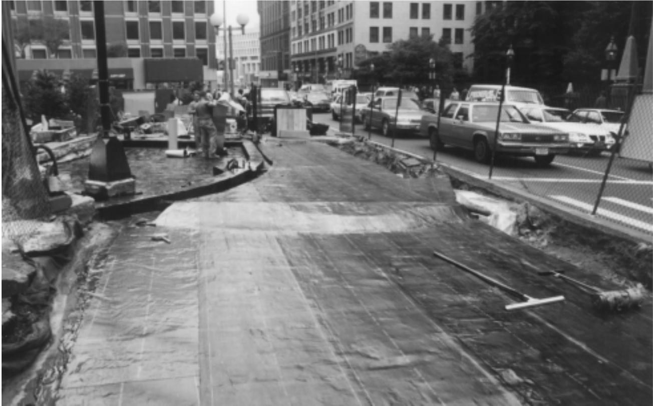
A self-adhered rubberized asphalt sheet membrane.
