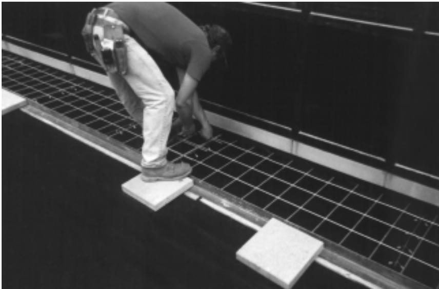
The membrane, insulation, and protection fabric are in place for this plaza installation. The welded wire mesh is installed prior to pouring concrete.
