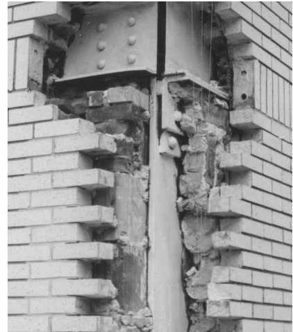
▲ Addressing the root causes of masonry distress avoids wasting time and money on duplicate repairs. Here, replacing rusting steel supports before rebuilding the face brick provides a long-lasting solution.
