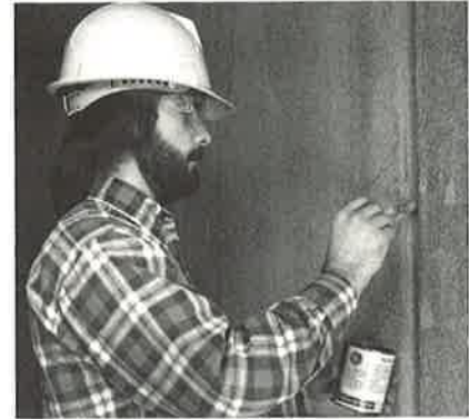
applying primer to a concrete substrate
