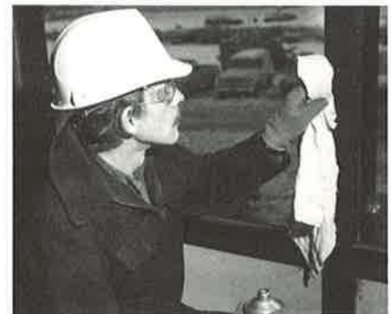
a white rag used to clean the substrate shows when it is too dirty to use
