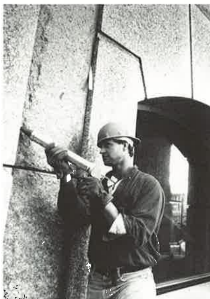
sealing a stone building
