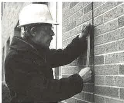
brushing the substrate will help remove loose particles that inhibit adhesion
