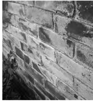
▲ Efflorescence.
