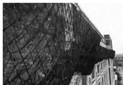
▲ Until permanent repairs are made, netting may be used to secure unstable terra cotta.
