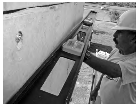
▲ To true the wall surface, the installer should level the insulation board, rather than build up base coat.
