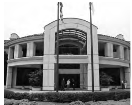
▲ Pfizer, Inc., North Maple Inn in Basking Ridge, New Jersey. Facade Rehabilitation.
