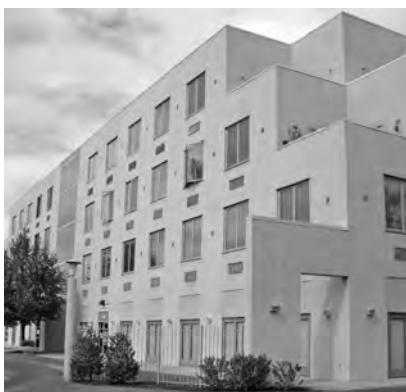
▲ Windsway Condominium in Norwalk, Connecticut. Water Infiltration Investigation.
