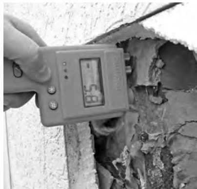
▲ Moisture meters may be used as part of an EIFS failure investigation.
