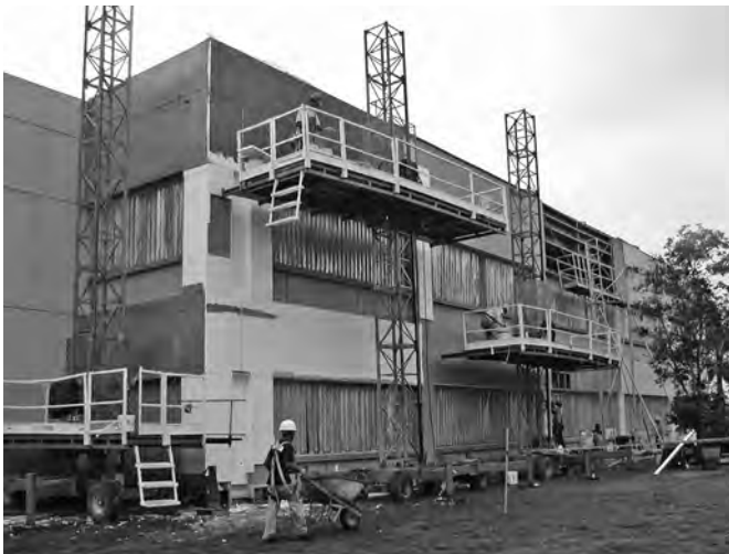
▲ For retrofit projects aiming to improve performance and update appearance, EIFS provides a practical option.
