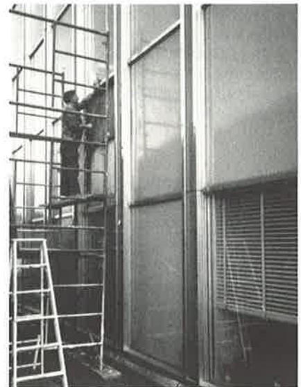
repairs to an aluminum curtain wall
