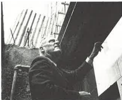
project architect Ted Babbitt inspects deteriorated steel beams
