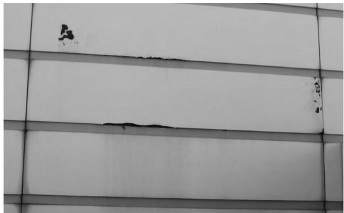
▲ Cladding design should encourage water to drain down the surface of the facade. Here, condensation has led to corrosion and premature degradation of the metal panel system.
