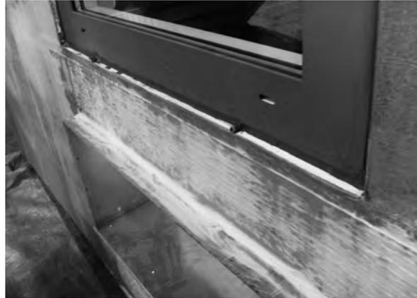
▲ Mockup of wall and window installation, showing fluid-applied waterproofing and weep tubes.
