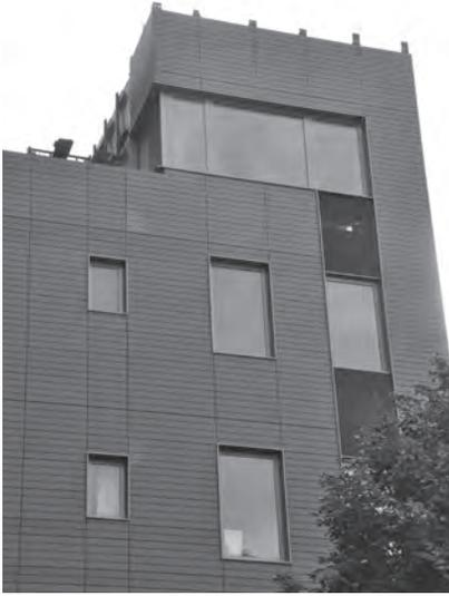
▲ Terra cotta facade system incorporating multi-layer water penetration protection.
