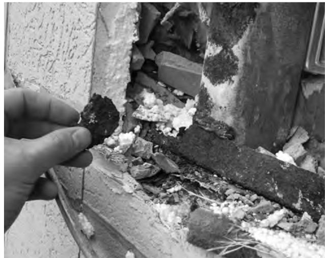
▲ Evidence of moisture damage at this face-sealed EIFS assembly includes corrosion, delamination, and mold.
