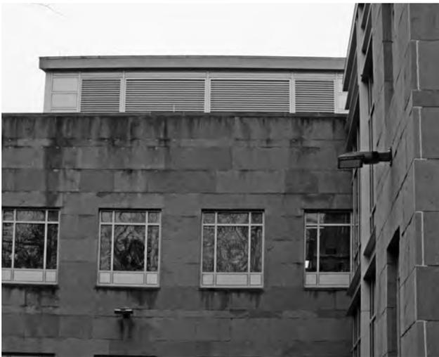
▲ Water washing down the face of this sandstone veneer facade has led to staining and algae growth.
