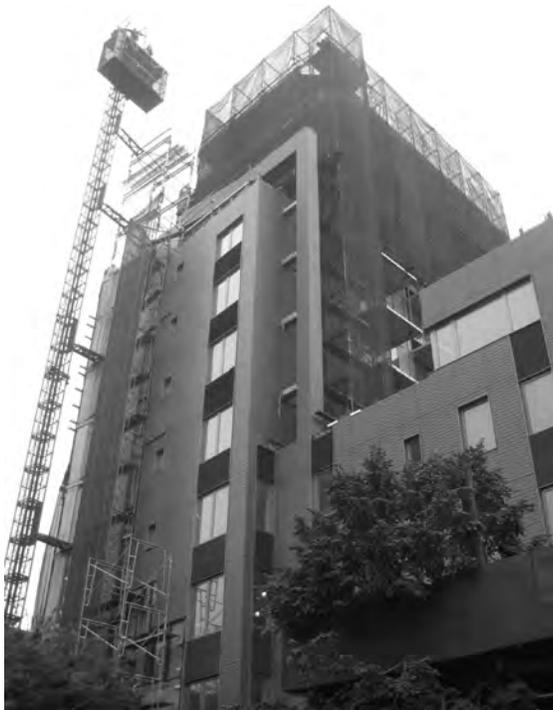
▲ Installation of a facade panel system that uses a rain screen approach to control moisture. Prime Architect: CetraRuddy Building Envelope Consultant: Hoffmann Architects, Inc.
