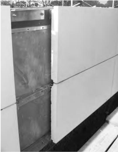
▲ A variety of cladding materials can be used with a rain screen design, including thin precast concrete veneer, pictured here.
