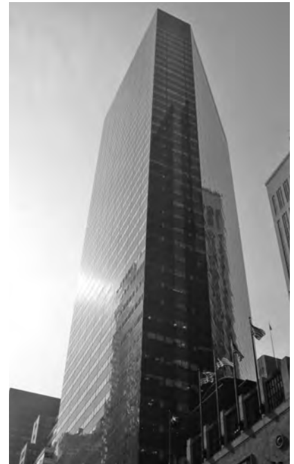
▲ Edward J. Minskoff Equities at 590 Madison Avenue in New York, New York. Glass/Granite Curtain Wall Repair.
