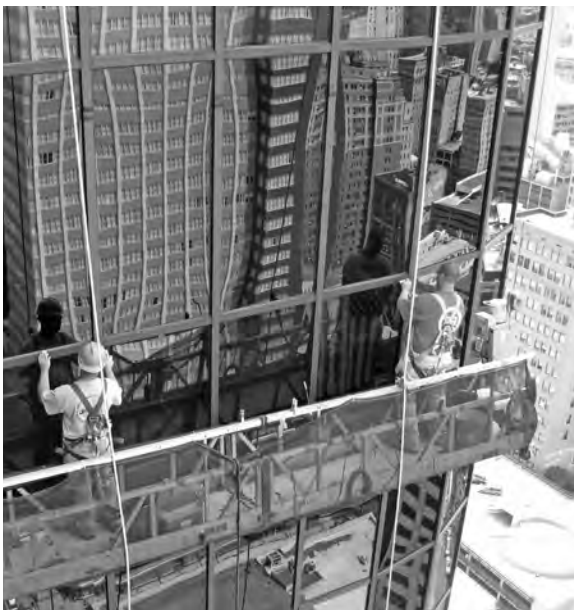
▲ Workers repair failed gaskets at a glass curtain wall high-rise.
