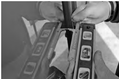
▲ Evaluation may include measurements of gasket hardness (top) and of glazing alignment (bottom).
