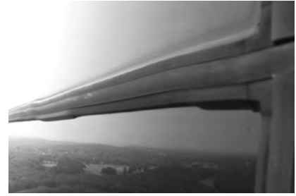
▲ Gaskets disengaged from glazing.
