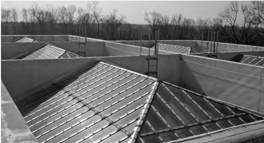
▲ An integral part of the balance of light and mass in many Modernist buildings, skylights are also notorious for leaks, condensation, and poor energy performance.
