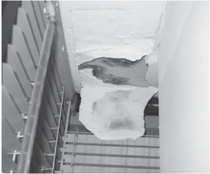
▲ Exterior investigation, rehabilitation, and expert witness services for an office complex.
