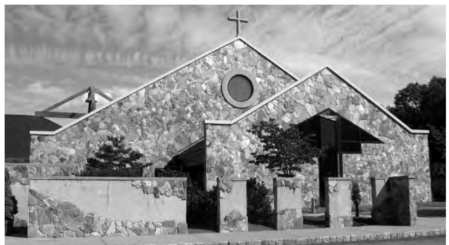
▲ Blessed Kateri Tekakwitha Parish in Sparta, New Jersey. Thin Stone Veneer and Roof Rehabilitation.
