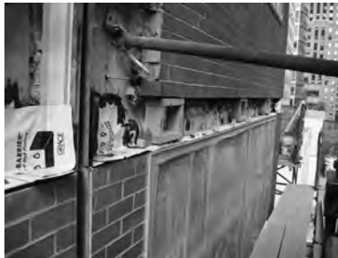
Installation of new flashing at window head.
