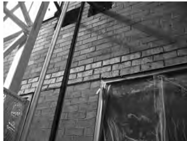
Reconstruction of brick exterior wall after flashing replacement.
