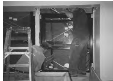
Installation of replacement windows.
