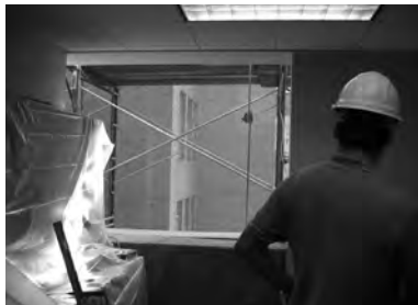
Window removed; wall opening ready for replacement window installation.
