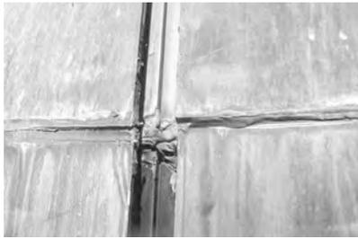
▲ More is not better: The use of too much sealant, especially one that is inappropriate for a particular joint application, will result in not only an unpleasant appearance but also premature sealant failure.
