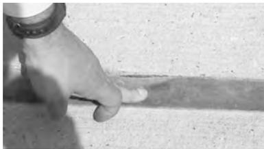
▲ Sealant failures at joints on horizontal surfaces such as this drive slab are typical in garages. Here, what may seem minor often leads to premature failure of parking decks and damage to tenant vehicles.
