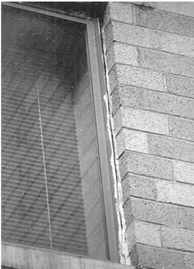
▲ Sealant failure at an aluminum-framed window. Aluminum expands and contracts nearly four times as much as brick masonry due to temperature changes. A sealant must be selected that will accommodate that movement.
