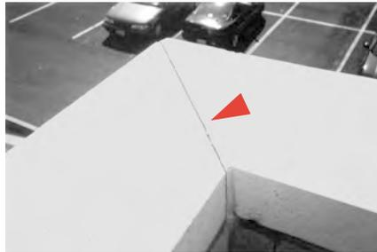
▲ Above left: When is sealant at the end of its useful life? When adhesive failure allows water to enter the wall through the coping. Above right: Adhesive failure along sealant joint of pilaster.
