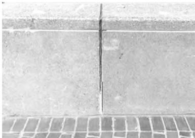
▲ At this plaza, sealant failures at perimeter walls and inadequately terminated base flashing could be allowing water to enter open joints.
