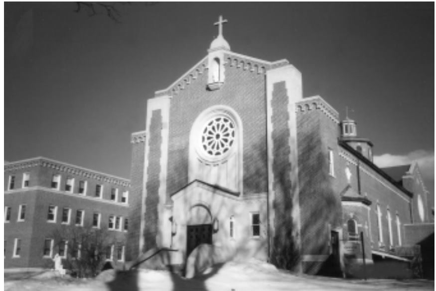
▲ Our Lady of Angels Motherhouse and Chapel Enfield, Connecticut. Hoffmann Architects cleaned the facades of existing water repellents to enable the brickwork to breathe.
