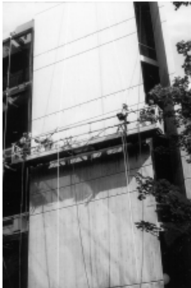
▲ Workers pressure wash the concrete façade of a corporate office building.
