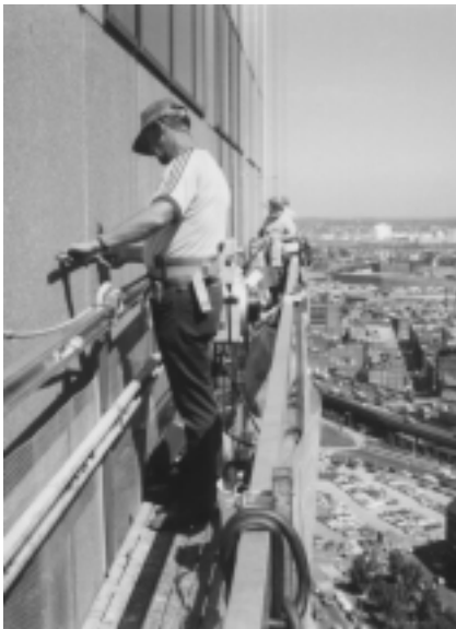
Thin-stone veneer being prepared for face-pinning.
