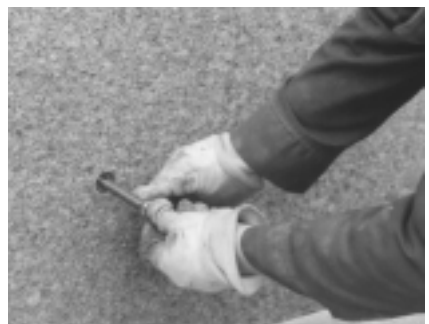
Step 3: Inserting the anchor rod with nut.
