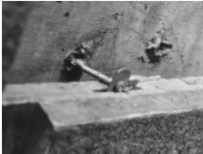
An anchor set in a slot in the top of a thin-stone panel.
