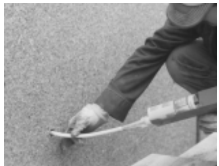
Step 2: Injecting the epoxy adhesive into the anchorage hole.
