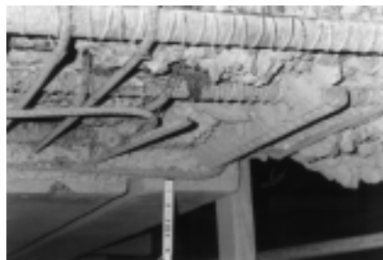
Deteriorated concrete is removed with hydro-demolition.
