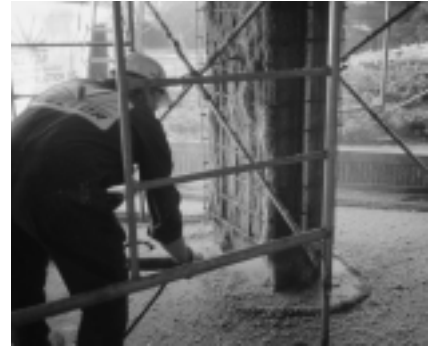
Applying sodium carbonate in preparation for re-alkalization.
