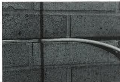
2. Installation of the backer rod.
