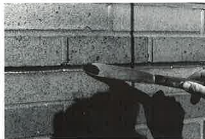
4. Sealant is tooled for a smooth finish.
