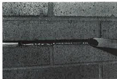
3. New sealant is applied.
