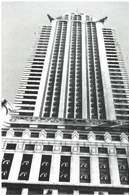
Glazed brick is an essential element of the Chrysler building's distinctive facade.
