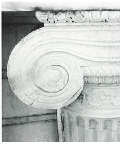
Detail of marble column showing deterioration of the capital. Note severe cracking in the volute.
