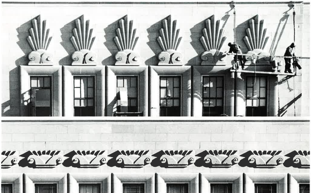
Restoration of limestone facade at Art Deco-style headquarters building.
