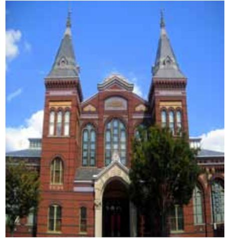
Despite a number of roof repairs, the building was plagued with leaks, some severe enough to warrant suspension of tarps from the rafters to protect exhibit halls below. Plaster ceilings sustained extensive water damage, and steel roof deck panels were badly corroded. The Smithsonian decided that it was time to determine the cause of the recurrent problems, and to resolve them.
