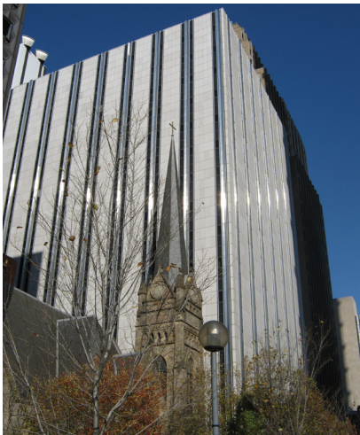
▲ AT&T / Koppers Tower , Pittsburgh, Penn., BBI Ordinance 9-2004 Inspection and Testing.
