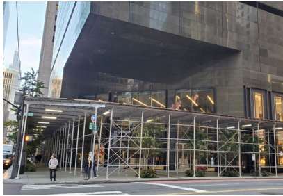
▲ Sidewalk sheds protect until repairs are done.
