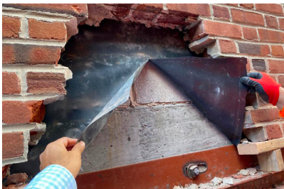
▲ NYC now requires cavity wall probes.
