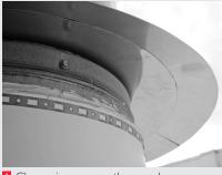
Clamp rings secure the membrane around circular penetrations.
