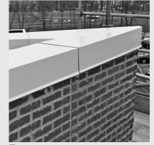
Parapet copings prevent water infiltration that can migrate under the roof membrane.
