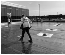
Electric leak detection is a non-invasive way to pinpoint breaches in the membrane.
