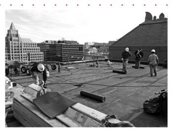
A Installation of a replacement modified bitumen roof (MBR) assembly provides durable long-term protection for this cultural institution.
