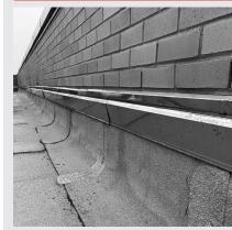
Metal counterflashing protects the upturned membrane edge at parapet walls.
