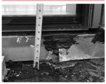
Low curbs and thresholds pose a challenge when insulation height must be augmented.
