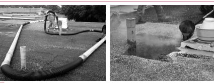
A Prior to installation of a recover system over an MBR assembly, loose granules in the existing cap sheet must be removed (*left*) or embedded in an asphalt flood coat (*right*).
