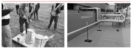
Two-component reinforced liquid resin recover systems, such as PMMA, cost more and require on-site mixing (*left*) but provide a seamless solution for complex roof areas (*right*).
