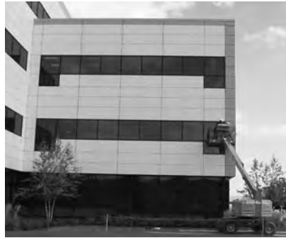
▲ Leak investigation at this steel panel facade pointed to faulty installation practices.
