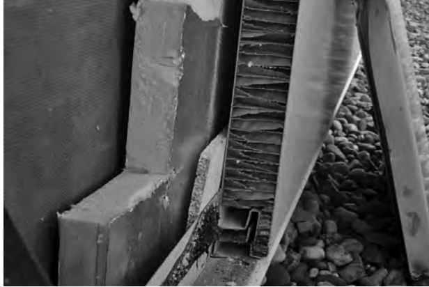
A Installed in the 1990s, this metal cladding system consists of painted steel composite panels with a paper honeycomb core. Rigid insulation, inboard of the panels, provides thermal resistance.
