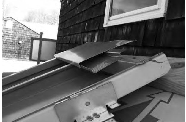
A This aluminum standing-seam roof system is installed over ice dam membrane, as well as stiffening ribs at the flat of each panel to minimize oil canning and telegraphing of structural members.
