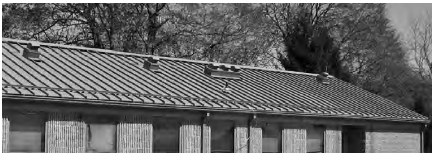
▲ For this military training camp, standing-seam aluminum roofs with a high-performance resin coating met fast-track project demands, while offering durability in the harsh seaside climate.
