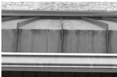
A Discoloration and staining
