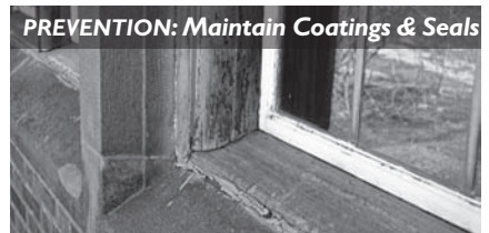
Freeze-Thaw and Salt Damage
