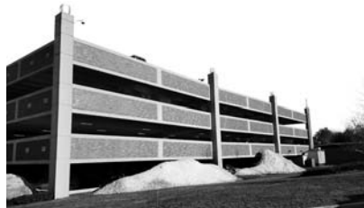
▲ Lahey Clinic Hospital in Burlington, Massachusetts. Parking Garage Investigation and Weather Damage Rehabilitation.
