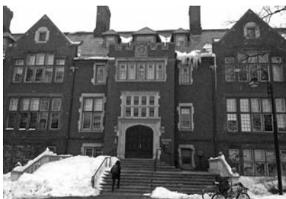
▲ Mount Holyoke College in South Hadley, Massachusetts. Exterior Envelope Assessment of 20 Buildings.
