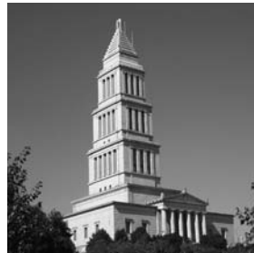
▲ Washington Masonic Memorial , Alexandria, Virginia, Earthquake Damage Evaluation.
