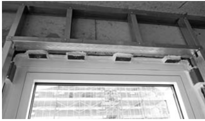
▲ High-efficiency details, such as warm spacers at window assemblies, prevent heat loss/gain by providing a thermal break at conductive materials, like metal-to-metal connections.
