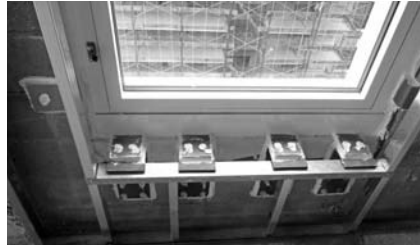
▲ High-efficiency details, such as warm spacers at window assemblies, prevent heat loss/gain by providing a thermal break at conductive materials, like metal-to-metal connections.
