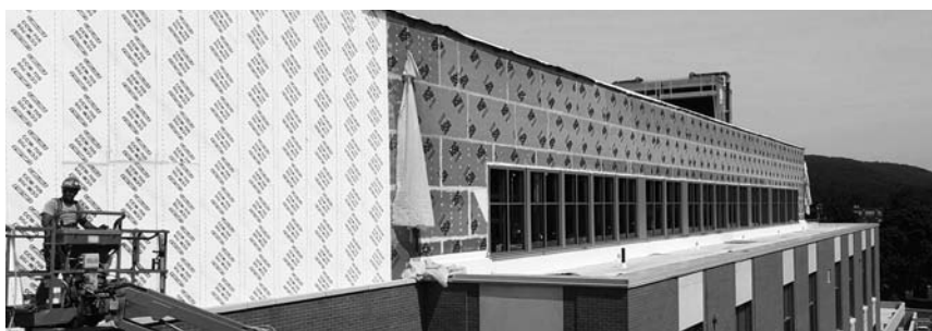
▲ At the top level of this energy-efficient building, an adhered air barrier provides the primary weather protection for a metal panel cladding system, to be installed.
