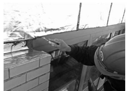
▲ A technician repairs a penetration in an air and vapor barrier system.
