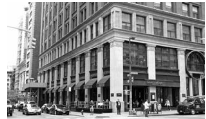
225 Park Avenue South , New York, New York, Building Envelope Consultation.
