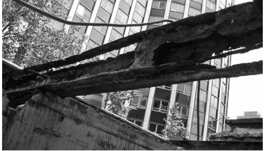
▲ At street level ( top left ), the sidewalk appears to be in good condition. In the vault below ( bottom left ), masonry arches show their age but seem structurally stable. Masonry removal, however, shows how badly deteriorated the embedded steel really can be ( above ).
