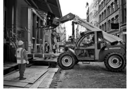
▲ Historic granite slabs are retained for reinstallation after vault rehabilitation.
