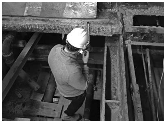
A An engineer investigates structural slab conditions at a partially deconstructed sidewalk vault.
