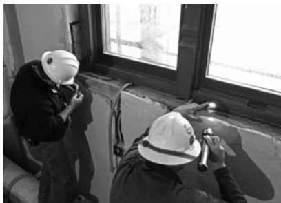
▲ Water infiltration field testing involves close analysis of frames and wall openings.
