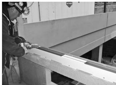
▲ Sealant is applied in preparation for energy-efficient glazing installation.
