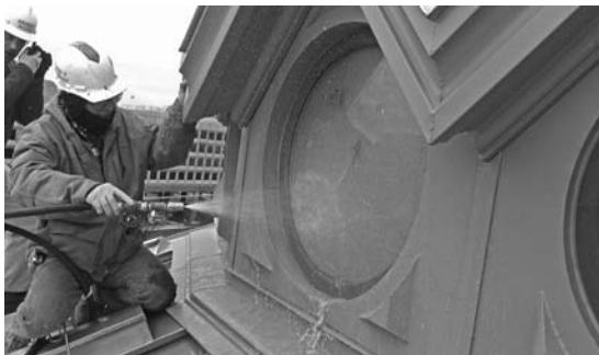
▲ Static and dynamic water penetration tests confirm the window assembly's conformance with design specifications.
