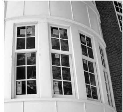
▲ High-performance replacement windows ( right ) resolve thermal inefficiencies and leaks that the retrofitted storm windows ( left ) at this historic building failed to adequately address.
