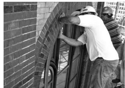
▲ Trim installation completes a custom historic window replacement.
