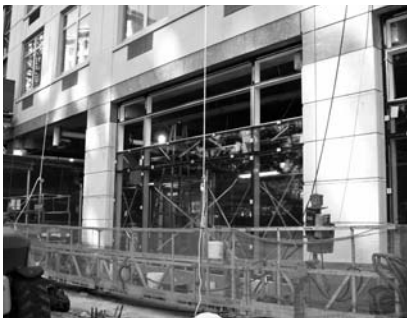
▲ Building codes specify glazing requirements for solar heat gain and thermal transfer.
